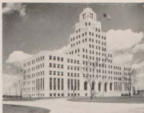
Staley Administration Building
