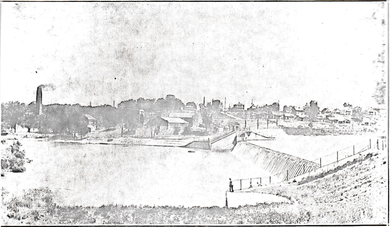
WATERWORKS AND DAM IN 1929
