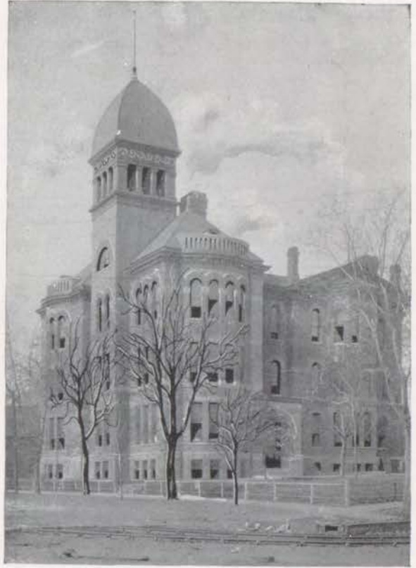
4—H. S. Building after two additions— Present Departmental School D. H. S. of 1895-1911
