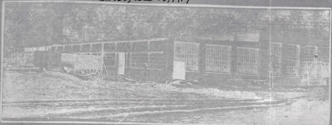
First unit of three for which foundations have been laid, in the Comet track tract. The total cost of the factory is to be $351,000. The Hoffman Construction Co. of Terre Haute and Evansville has the contract, and the first unit was to be completed March 2, but probably will be delayed somewhat because of the early severe weather this year. —Photo by Wagon Studio.
