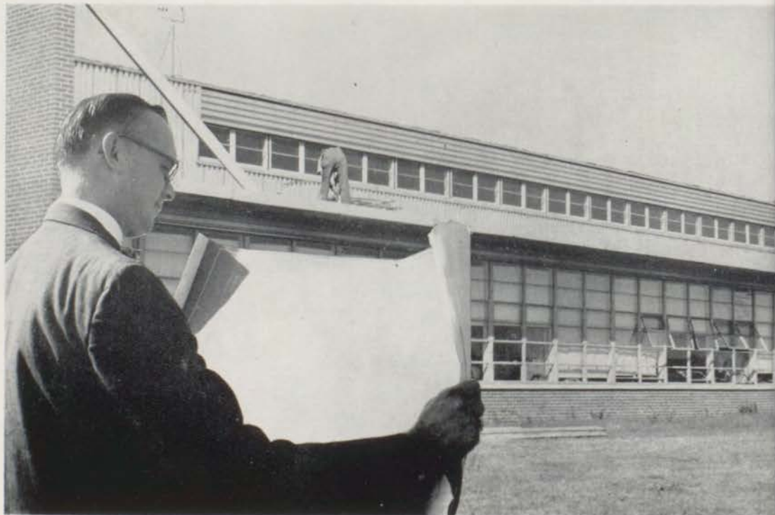
Construction of second story addition to south wing of building was the big architectural change this year.
