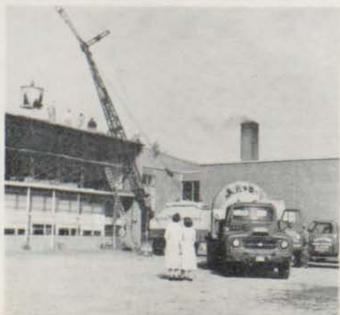
When completed, Junior High made immediate use of new addition.
