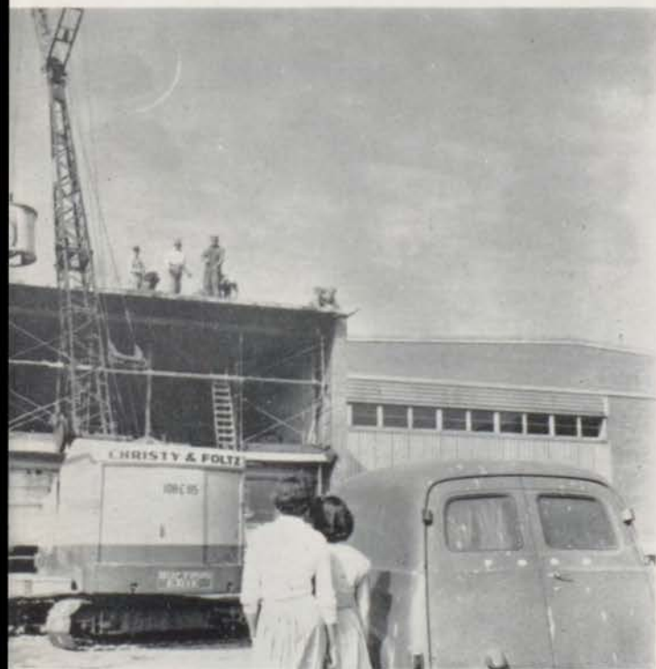
Observing construction work is favorite noon-time activity.
