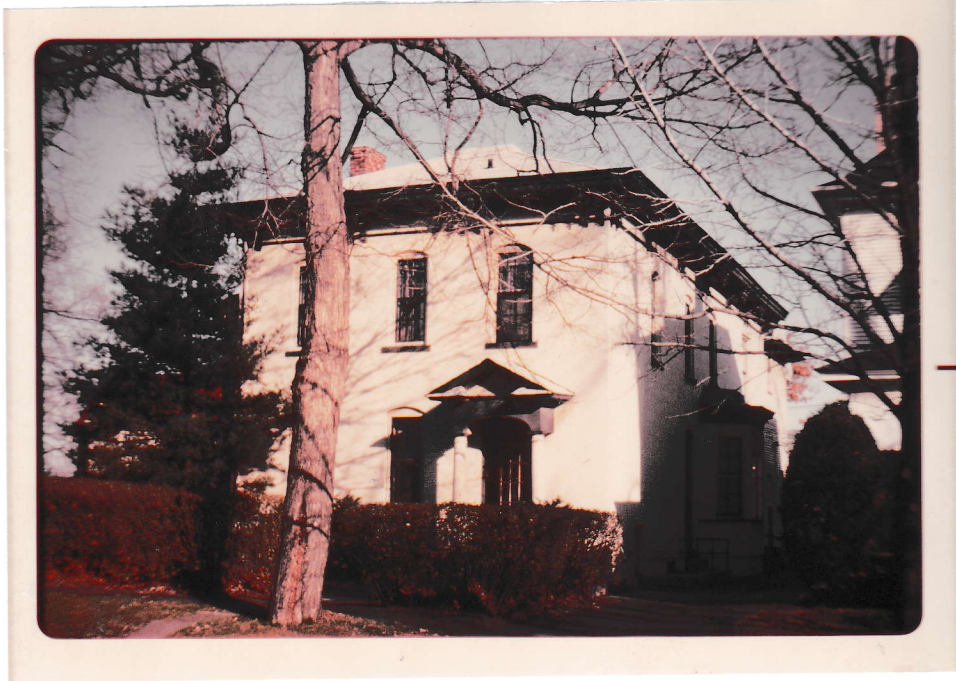
West side (front) of house
